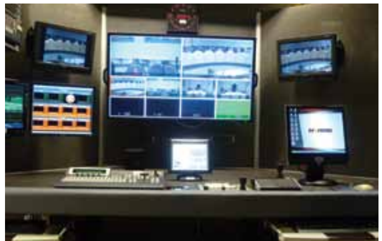
Nunavut legislature control room showing the Panasonic AV-HS-450 Switcher, Vinten control panel, Inscribe CG and Sharp multi view LCD screen.
